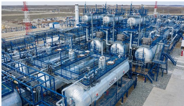
Oil treatment package for Tazovsky oil, gas and gas condensate field of Gazpromneft-Development, LLC Oil capacity, t/year: up to 2,200,000; Liquid capacity, t/year: up to 6,000,000; GOR, nm 3 /t: no more than 10
